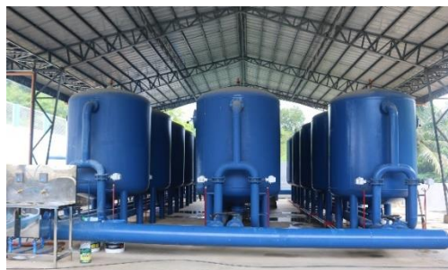
Water Treatment Plant in Takdog
