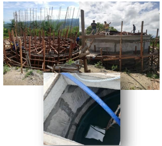
➤ Construction of Cayam Napo Reservoir
